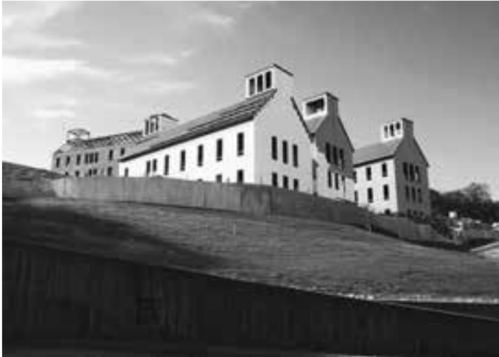
Current construction of the Hillside Campus
