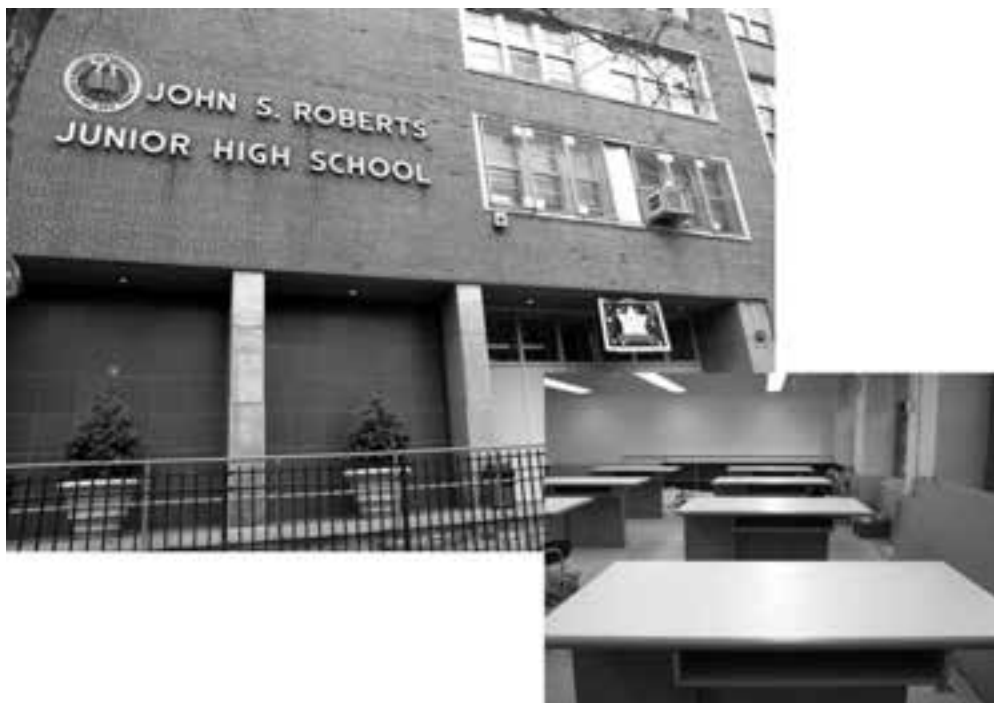
Renovations to the former graphics lab in J.S. Roberts Junior High School were near completion in early December.
