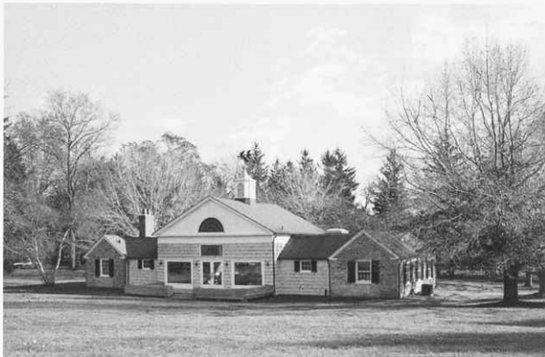
Back view of Banbury Conference Center
