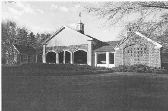
Front view of Banbury Conference Center.
